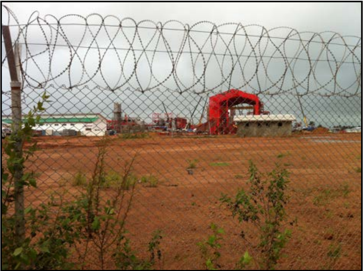
Figure 7: Factory site in September 2013. Fenced in with barbed wire. The central red building, the Cane Mill remained without a rooftop, Source: Photo Samuel Lustenberger.
